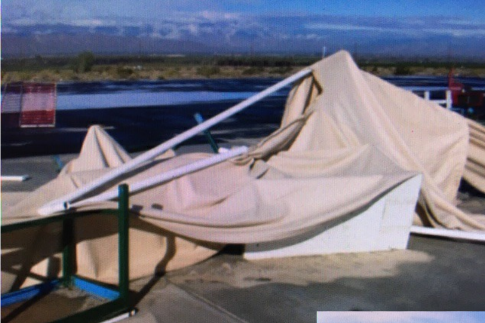
Wind and flood damage at our field in past years.
